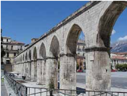
Sulmona, Aqueduct (13 th century)
